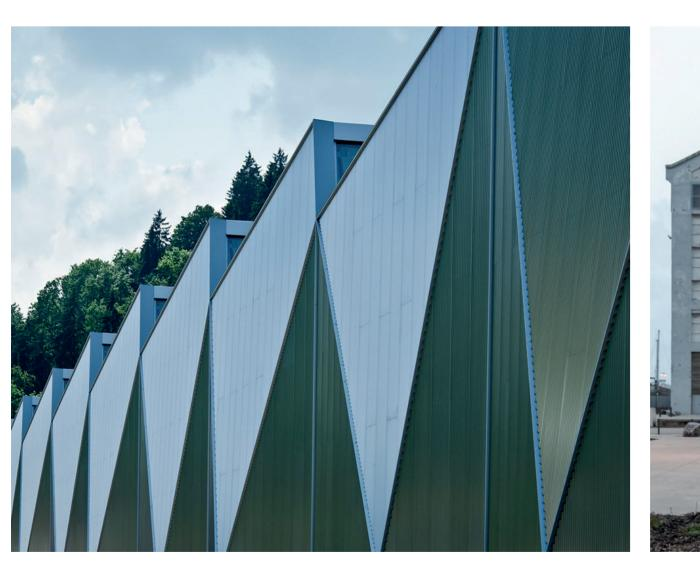
Cladding might be arranged in an Simple pitched roof forms angular format to create texture and interest. North facing rooflights allow natural light to penetrate the plant and limit the requirement for artificial lighting.
